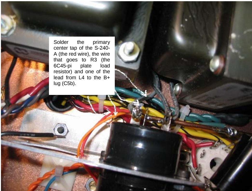
Figure 45. Wiring the B+ (C 5b ).
